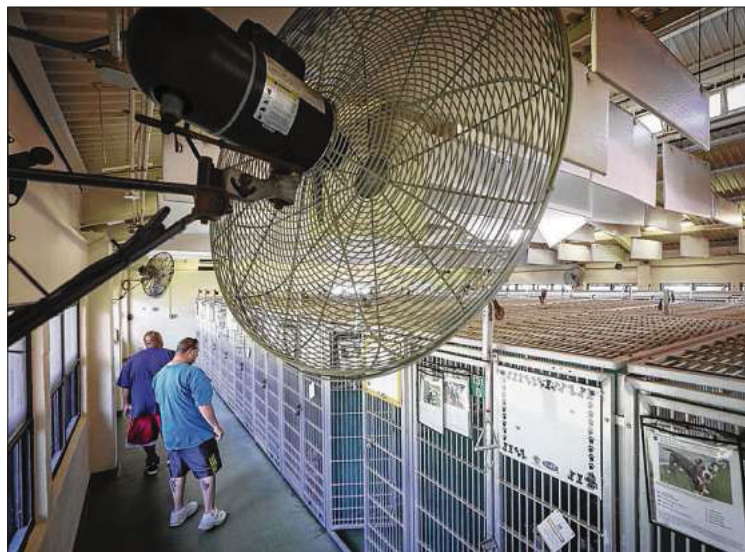
Overhead fans circulate the air in a kennel at Palm Beach County Animal Care and Control. "It is a brutal summer," said director Dianne Sauve. "These fans run 24/7. The kennels were never designed to have air conditioning."
